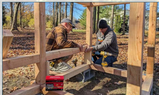
Community Composting Facility Starting
